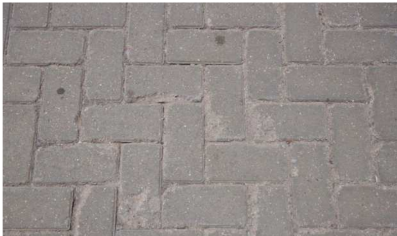
The severe erosion of the Strand pavers (left) is a marked contrast to the Mouille Point pavers (right) which show minimal erosion after double the lifespan
