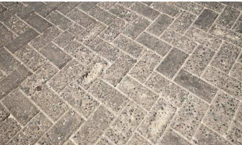
The severe erosion of the Strand pavers (left) is a marked contrast to the Mouille Point pavers (right) which show minimal erosion after double the lifespan
