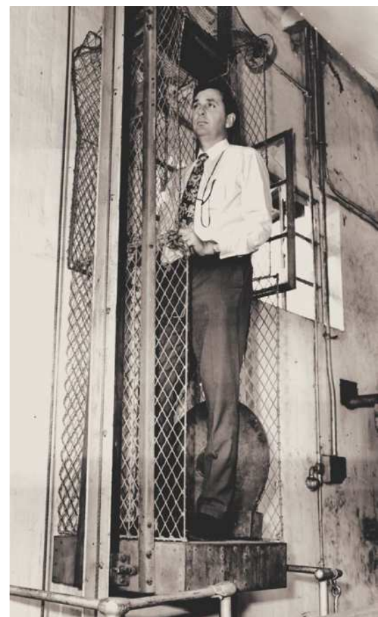
Figure 10 Operator on an internal man-lift, pulling up and down on a rope, assisted by a counterweight system
