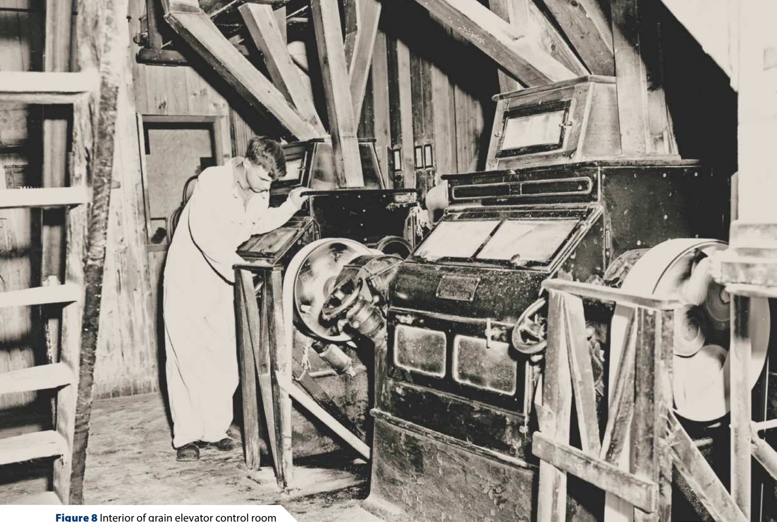
Figure 8 Interior of grain elevator control room
