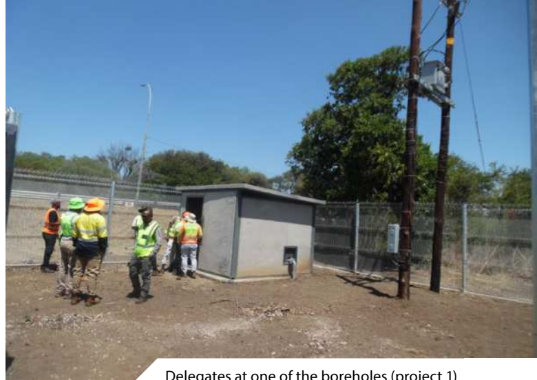
Delegates at one of the boreholes (project 1)
